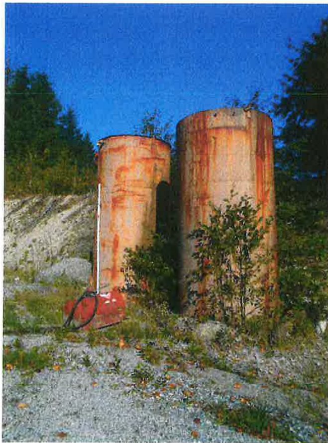
Figure 9. Water tanks and 55-gallon diesel AST along northern boundary.
