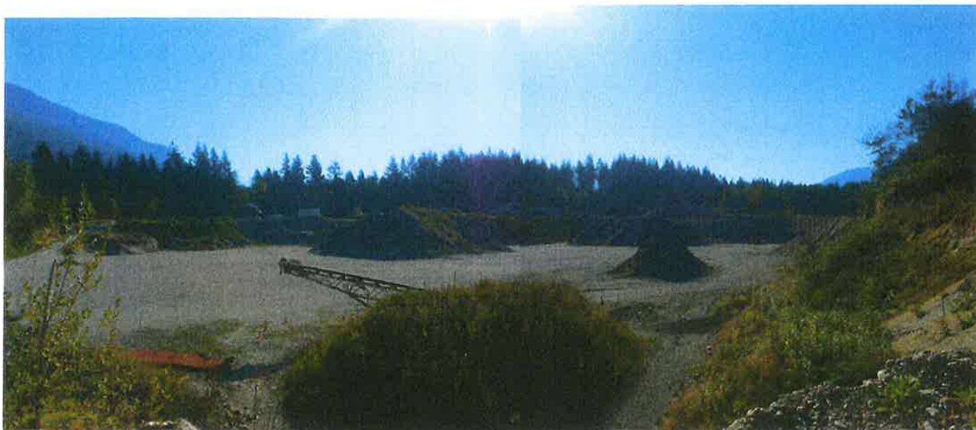
Figure 4. View of the property looking southeast from the top of the dike.
